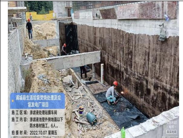
渗滤液池壁防渗铺贴
